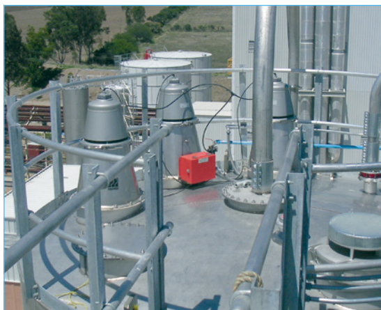
Stainless steel modular bin vents
